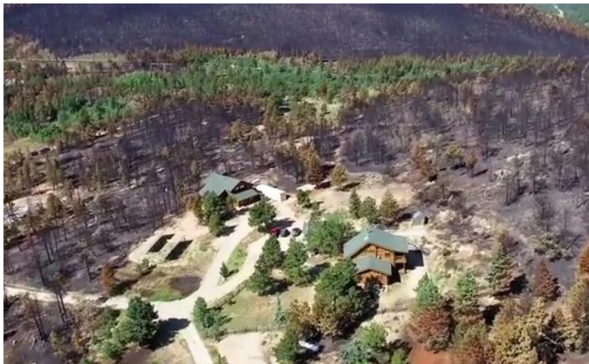
Defensible space allowed firefighters to protect this home during the 2016 Cold Springs Fire near Nederland, CO (source: Cold Springs Fire Success Stories from Wildfire Partners).
