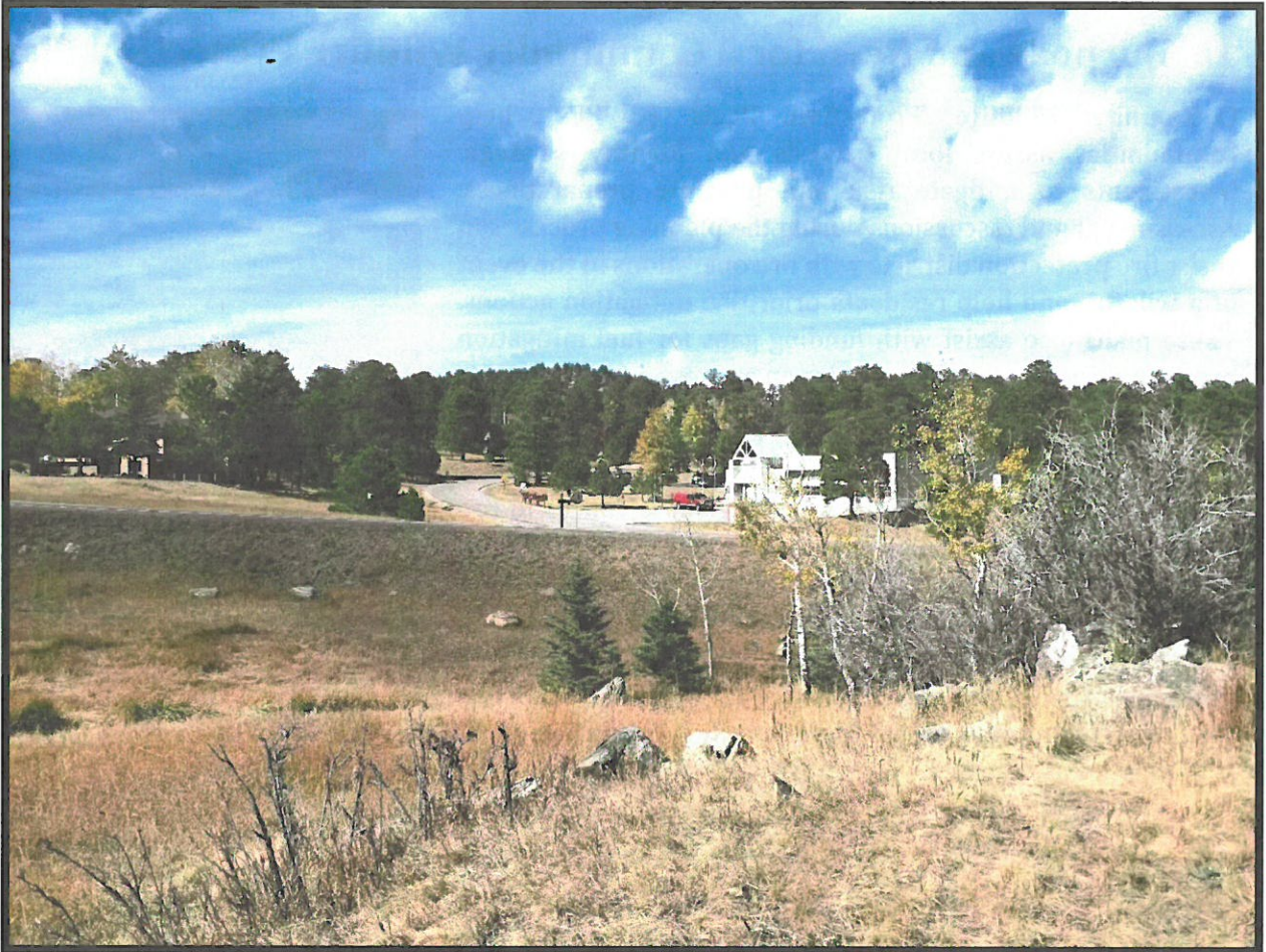
Headquarters for Genesee Fire Rescue—the local fire department that protects the Genesee Fire Protection District. Photo from the Forest Stewards Guild.
